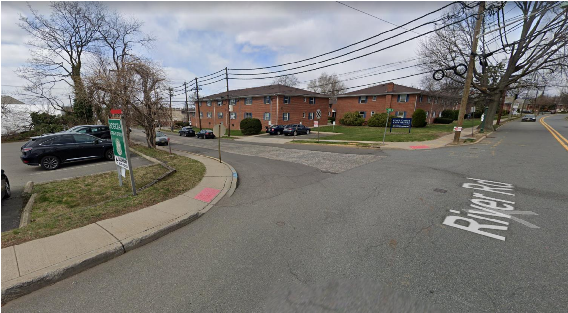
Photo 6: Existing intersection of River Road and Cross Street. Non compliant ADA ramp seen on the left hand side shall be replaced.
