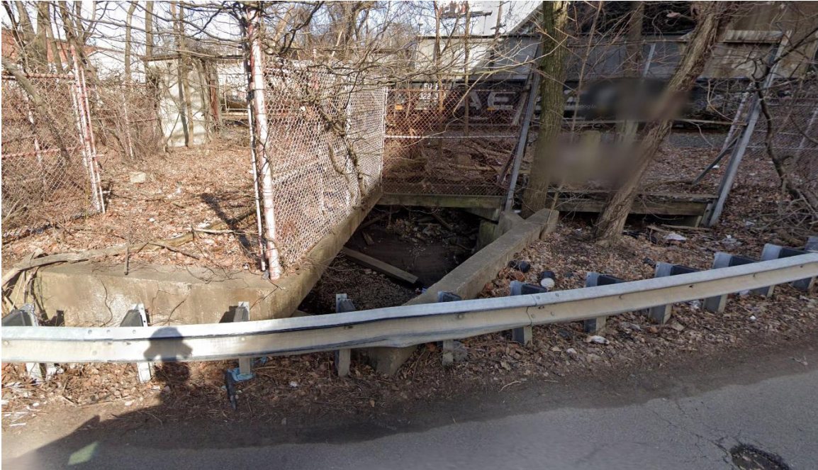
Photo 13: Location of the twin 60" RCP pipes that run under Industrial Way.
