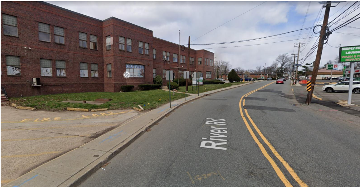
Photo 4: Looking northbound along River Road the existing frontage of the subject property can be seen.
