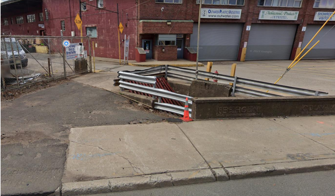
Photo 3: Beginning of the concrete chamber that runs throughout the site.
