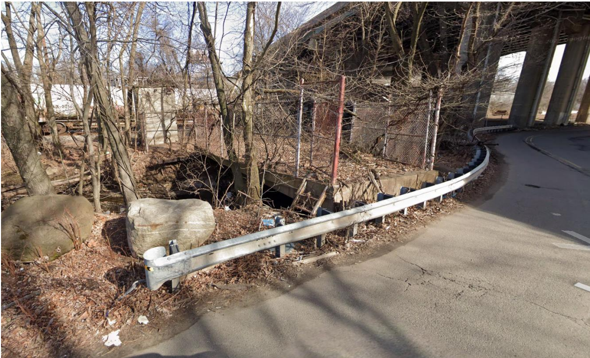
Photo 12: Existing parapet over the tributary to the Hackensack River. The undersized culvert is located directly north.
