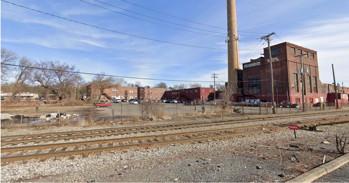
Photo 9: Looking East from Industrial Way at the west side of the site.
