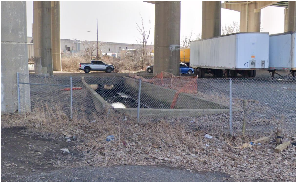
Photo 14: Open drainage concrete channel south of Industrial Way leading to the Hackensack River.
