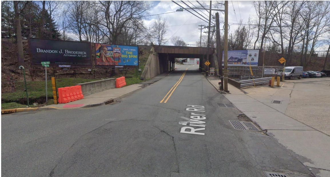
Photo 1: Looking southbound along River Road. The existing undersized culvert underneath River Road can be seen as well as the existing CSX railroad bridge.
