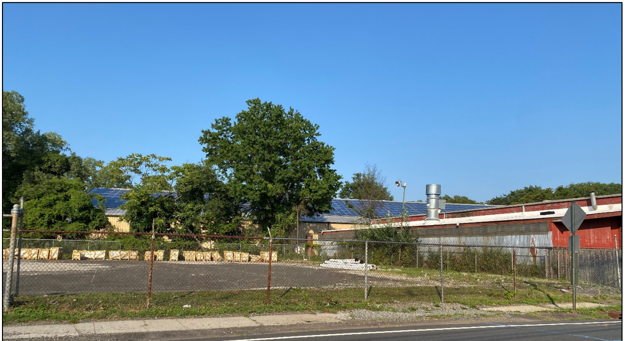
Looking across West Fort Lee Road towards east end of subject property
