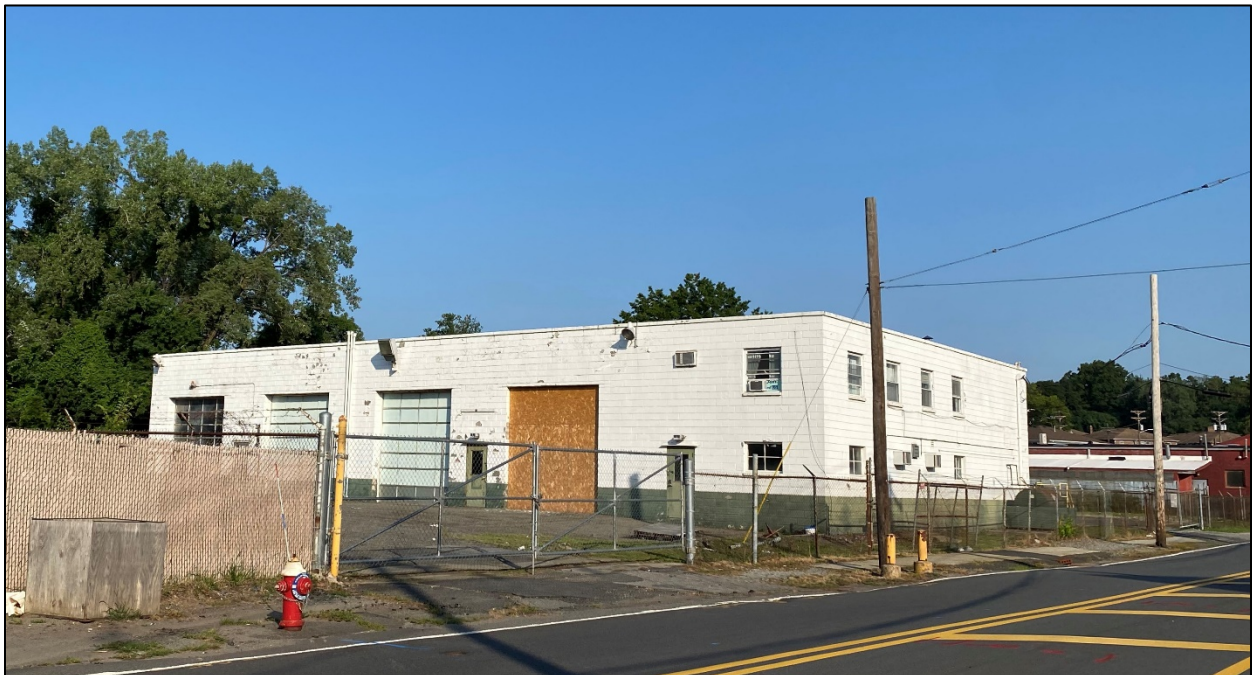
Looking west on Fort Lee Road across from subject property
