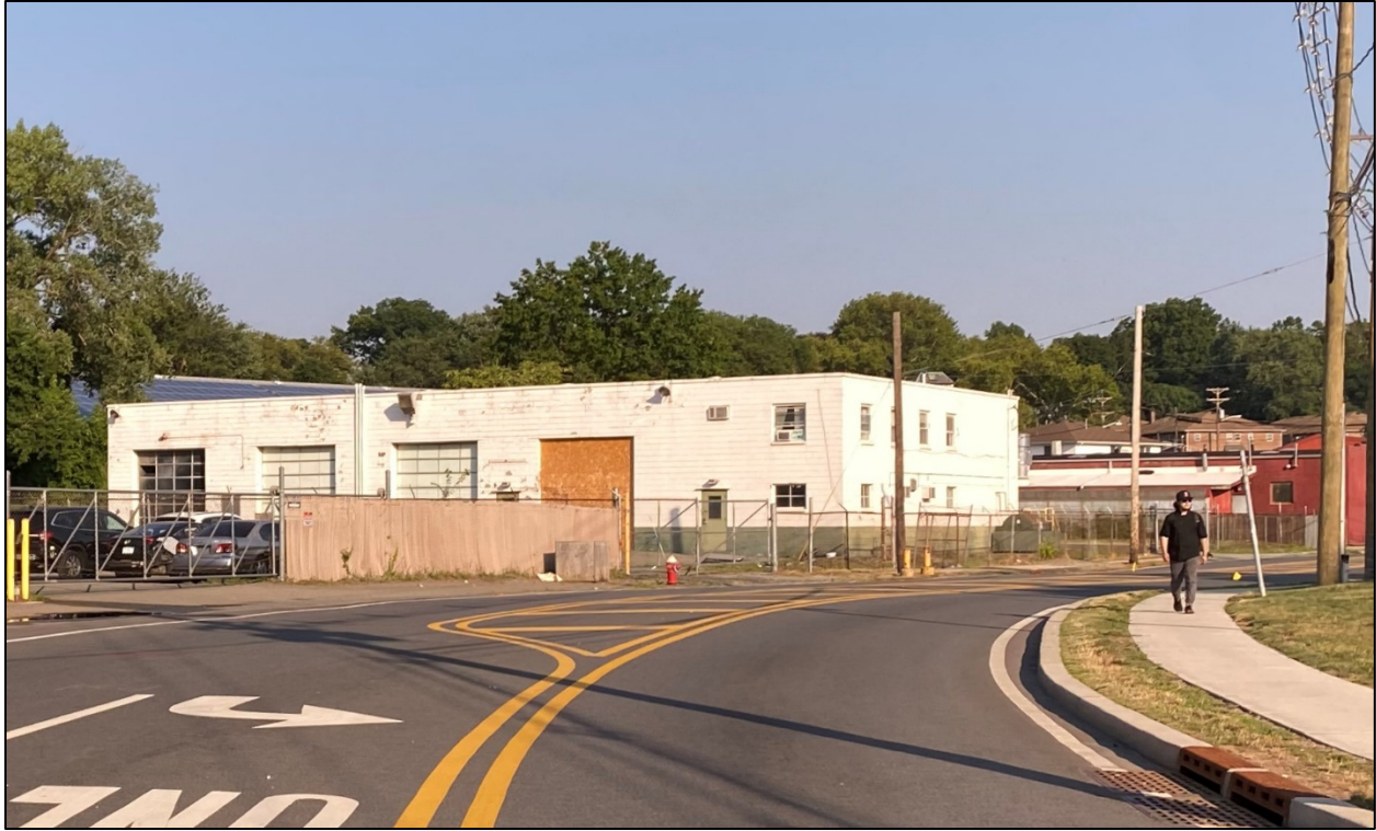
Looking east on West Fort Lee Road towards subject property
